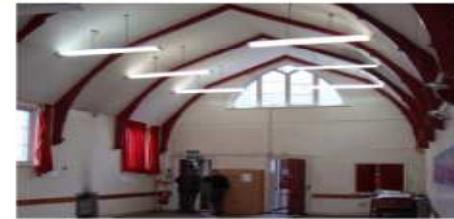
Internal view of existing hall
